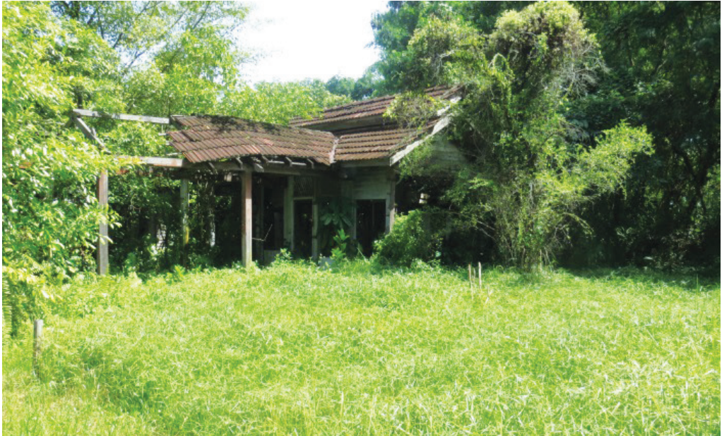
Gambar 24: Pelupusan kuarters lama Jalan Sanders di Ipoh, Perak Picture 24: Disposal of old quarters in Jalan Sanders in Ipoh, Perak
