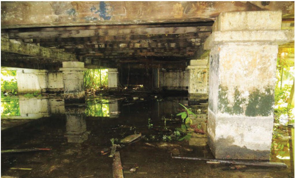
Gambar 25: Pelupusan kuarters lama Jalan Sanders di Ipoh, Perak Picture 25: Disposal of old quarters in Jalan Sanders in Ipoh, Perak
