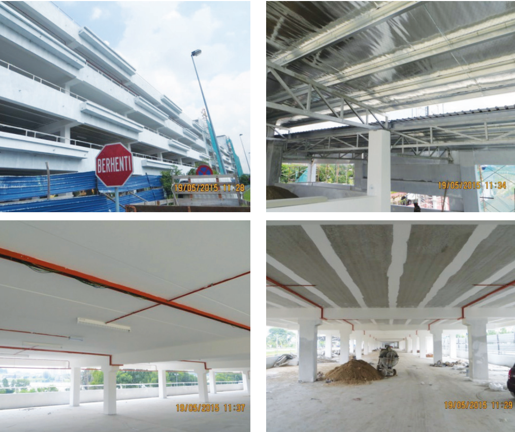
Gambar 23: Tempat Letak Kereta Bertingkat Park n Ride di Stesen Komuter Serdang yang hampir siap. Picture 23: Park n Ride multi-storey parking area at Serdang Komuter station which is near completion.
