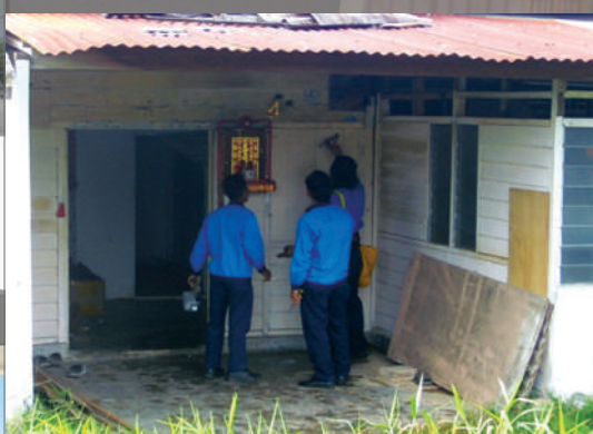
Petugas Tenaga Nasional Berhad (TNB) melaksanakan kerja pemotongan bekalan elektrik sebelum tindakan perobohan diambil. Tenaga Nasional Berhad (TNB) staff conducting operation to cut electricity supply before demolition works are implemented.
